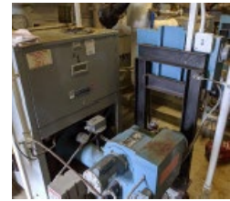
21 Figure 2-7. 22 Old boiler.
